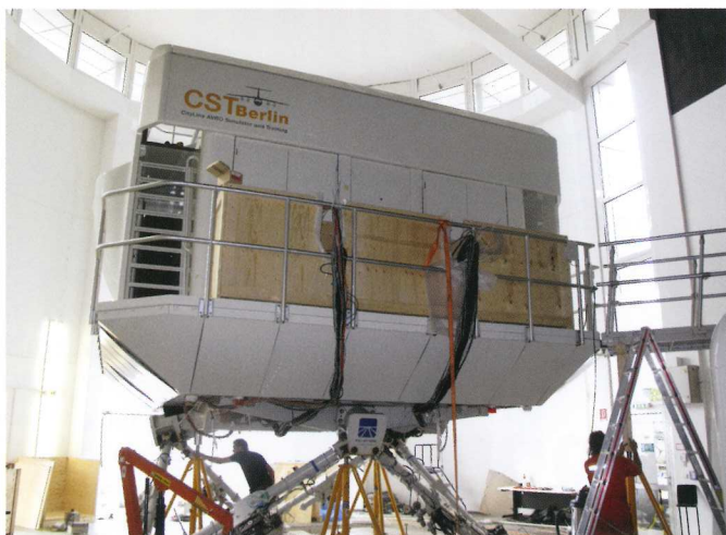
Piece by piece, the Avro RJ simulator is carefully dismantled.
